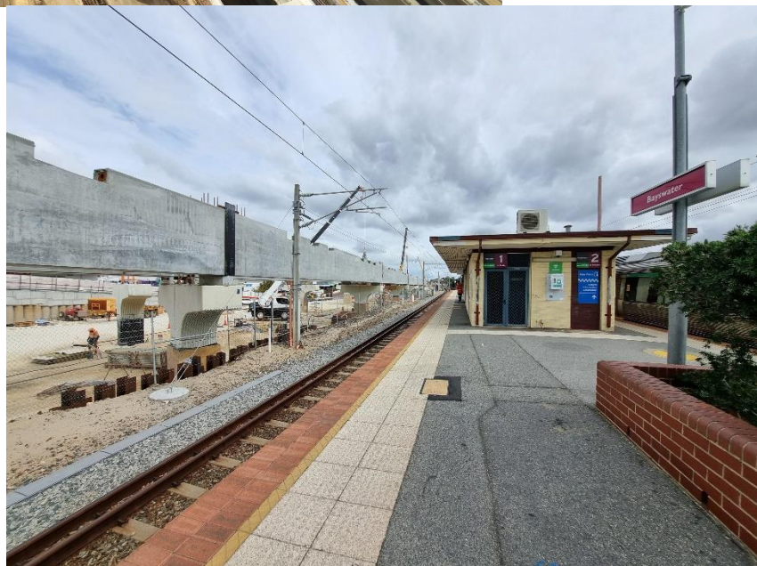
Below: close up of supports for the railway line which will be located to the south of the current track.
