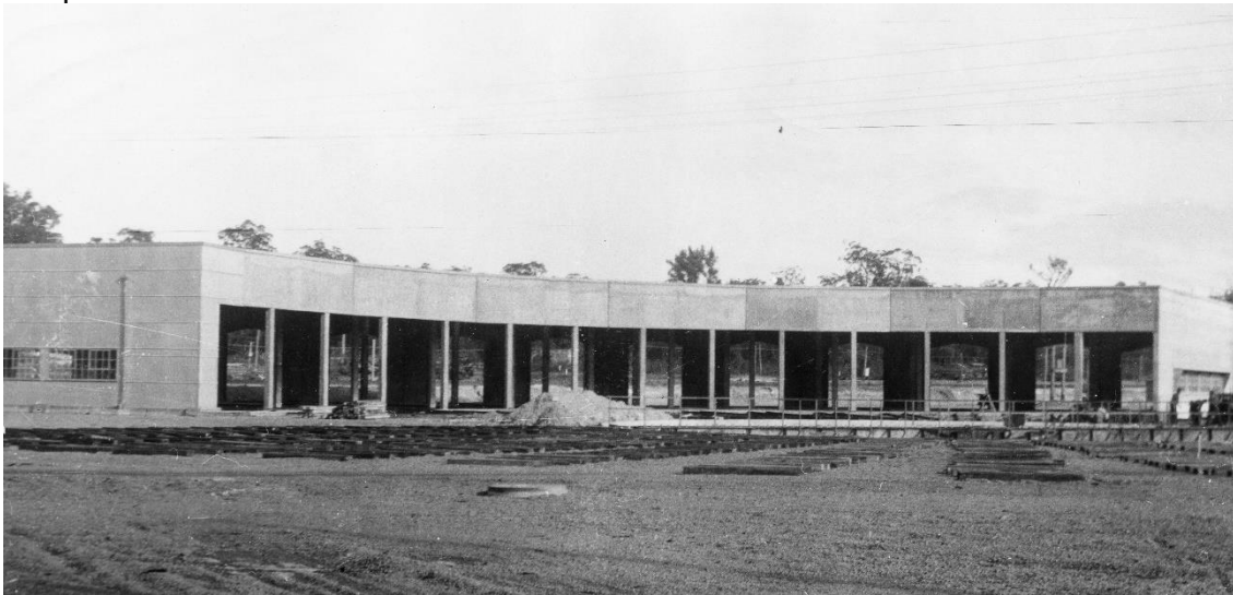
Collie Roundhouse under construction (RHWA Archives, P10048)
