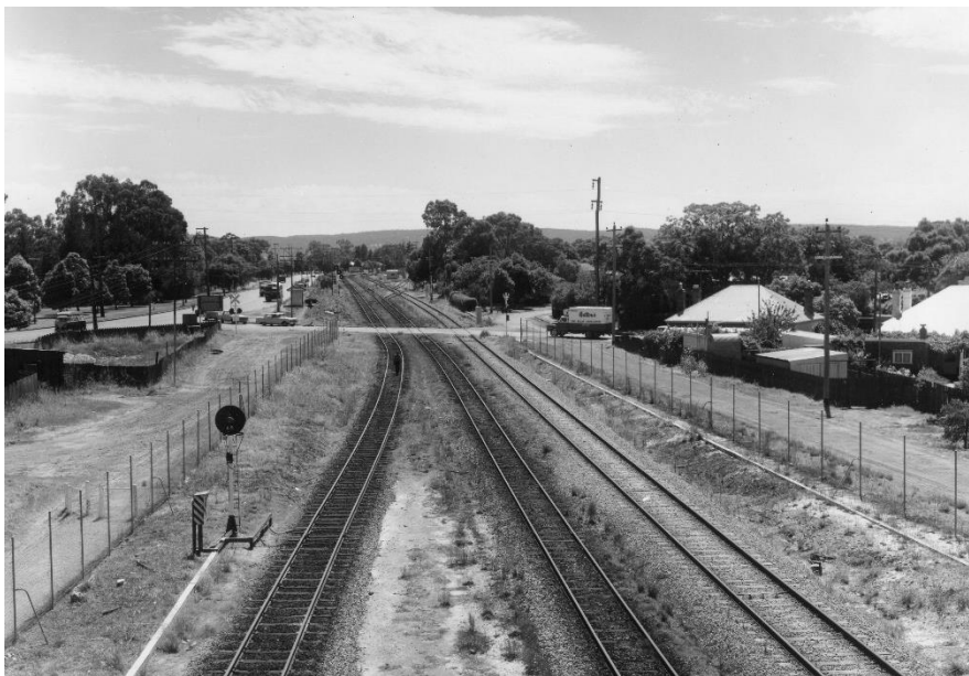
Trackwork and searchlight signal at East Guildford. View is from the footbridge looking east, new standard gauge track on the right.
