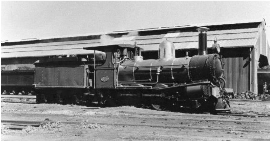
A 15 with a six-wheel tender, and a con rod missing. (P03199)
