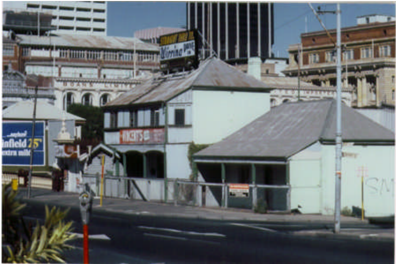
Second Clubrooms – No. 1 Beaufort Street Perth. On the corner of Beaufort Street bridge and Roe Street. December 1973 to July 1977
